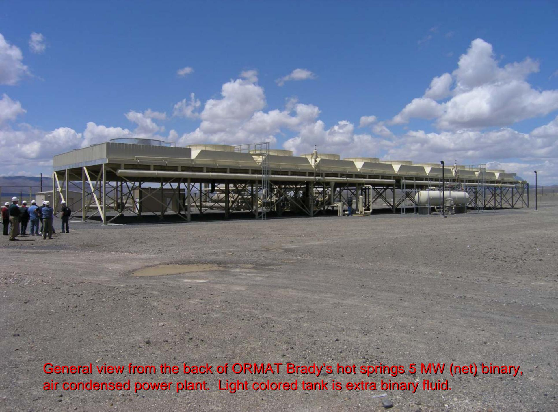
General view from the back of ORMAT Brady's hot springs 5 MW (net) binary, air condensed power plant. Light colored tank is extra binary fluid.
