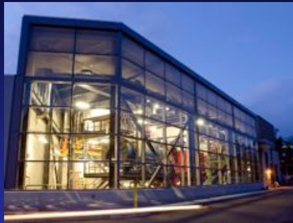
Middlebury College biomass boiler 2009; 5 MW thermal
