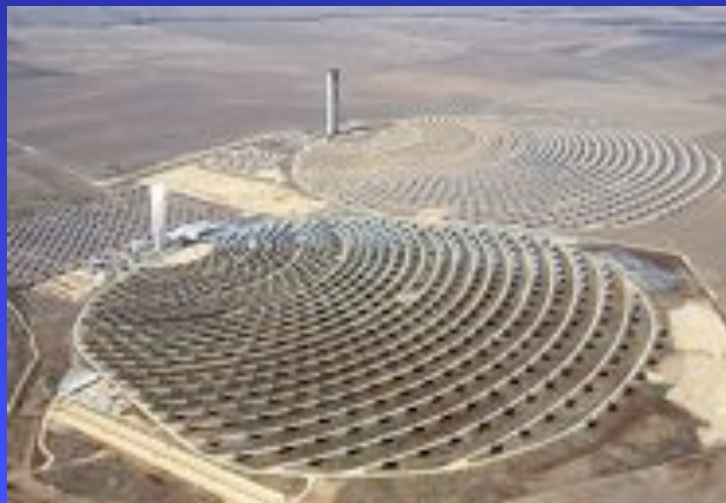
Concentrated solar-thermal, power towers (30 MW, Spain)
