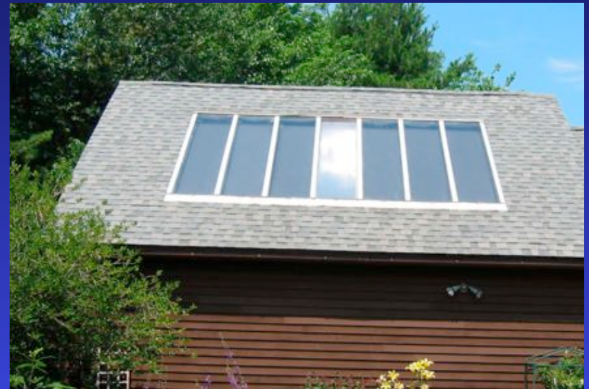
Active hot-water heating
