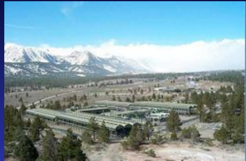
New: Mammoth Lakes, California 40-MW closed-cycle binary plant
