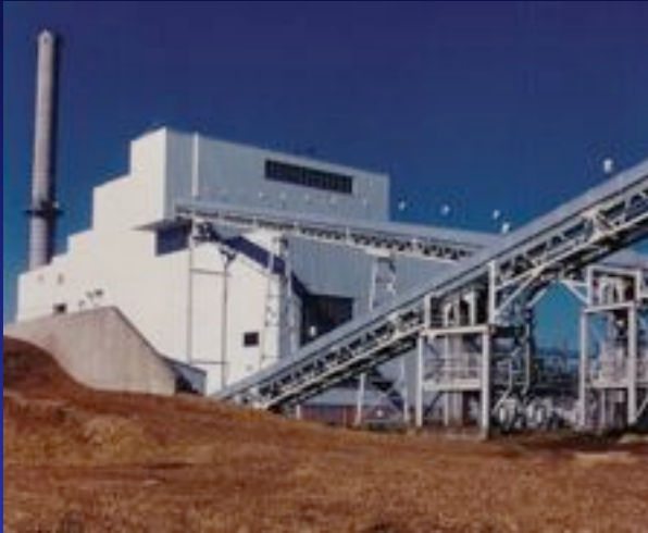
McNeil generating station, VT 1954; 54 MW
