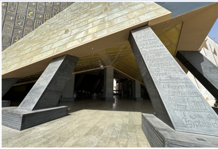
Entrance leads to a vast open-air atrium covered
