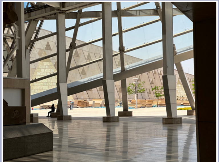
The museum is now open, but construction continues on the exhibits
